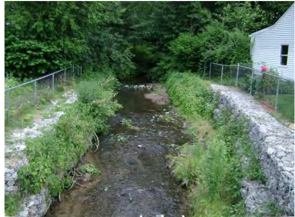
Figure 17b: Example of channelized stream with no pools in CB1. (Photo: RCE Water Resources Program)
